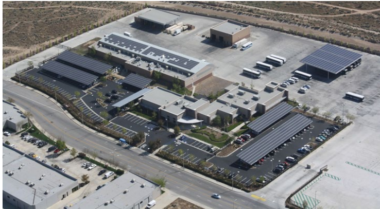
AVTA Lancaster Management and Operating Facility
