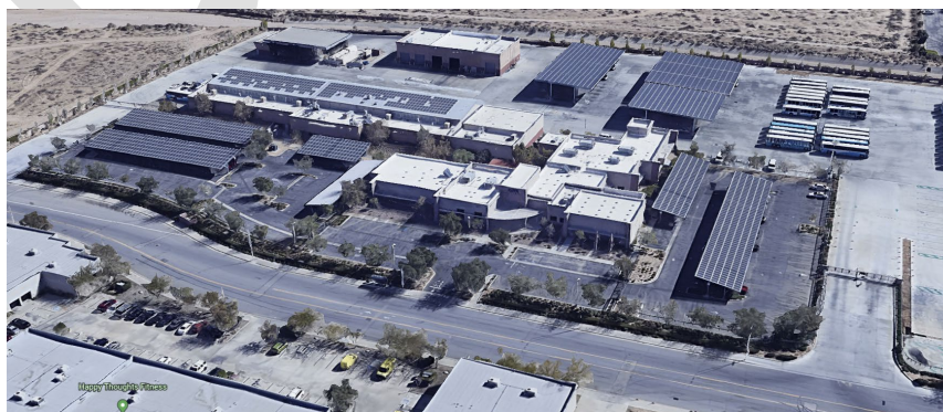
AVTA Lancaster Management and Operating Facility
