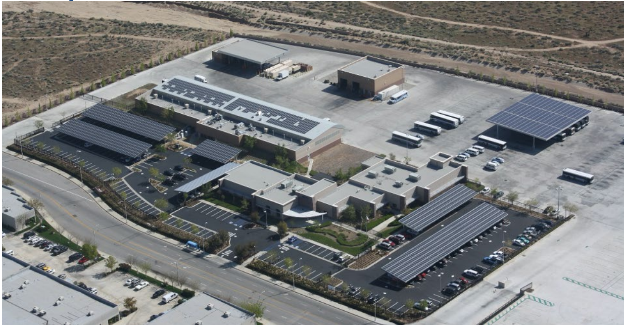
AVTA's Operations and Maintenance Headquarters, Lancaster, CA
