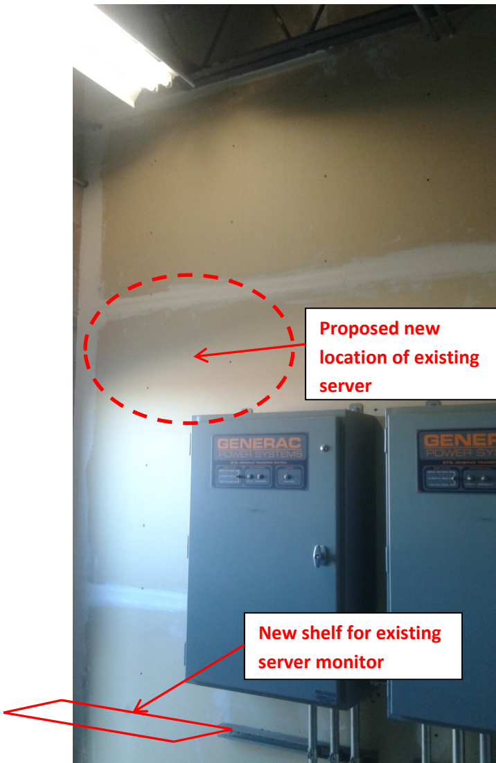
Photo 7 - East wall of Electrical Room
