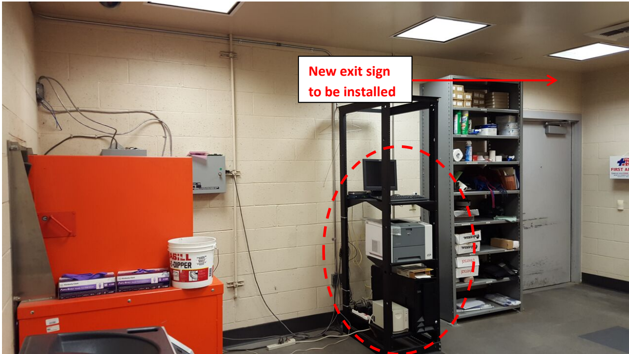
Photo 4 – Server (circled) to be relocated to existing Electrical Room by AVTA (see Photo 7)
