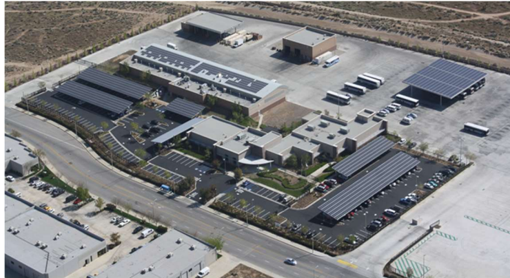
AVTA Lancaster Management and Operating Facility
